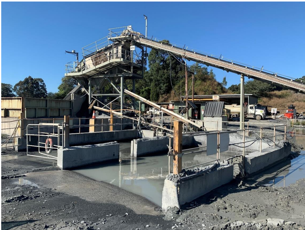
Washplant and wedge pit
