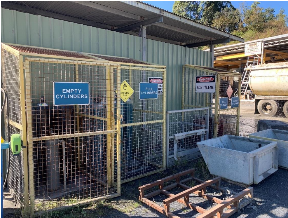
Secure storage available for dangerous goods, unlocked at the time of audit
